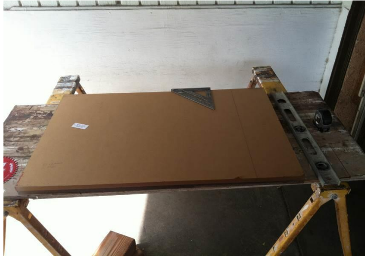
FIGURE 9. Working table preparations for marking required measurements for wall cuts.
