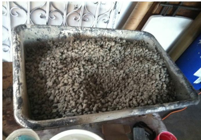
FIGURE 40. Concrete mixture with sufficient Portland cement to coat the aggregate.
