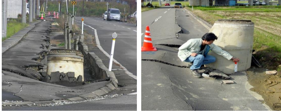
FIGURE 4. Flotation of sewage lines during 2004 Chuetsu earthquake.
