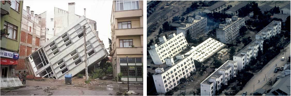
FIGURE 2. Bearing capacity failure due to differential settlement. (left) 1999 Kocaeli earthquake; (right) 1964 Niigata earthquake.
