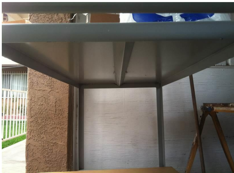
FIGURE 20. Bottom shelves reinforced with steel beams.
