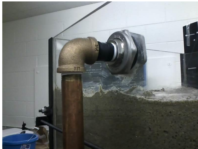
FIGURE 52. Overflow pipe connected to wall fitting.
