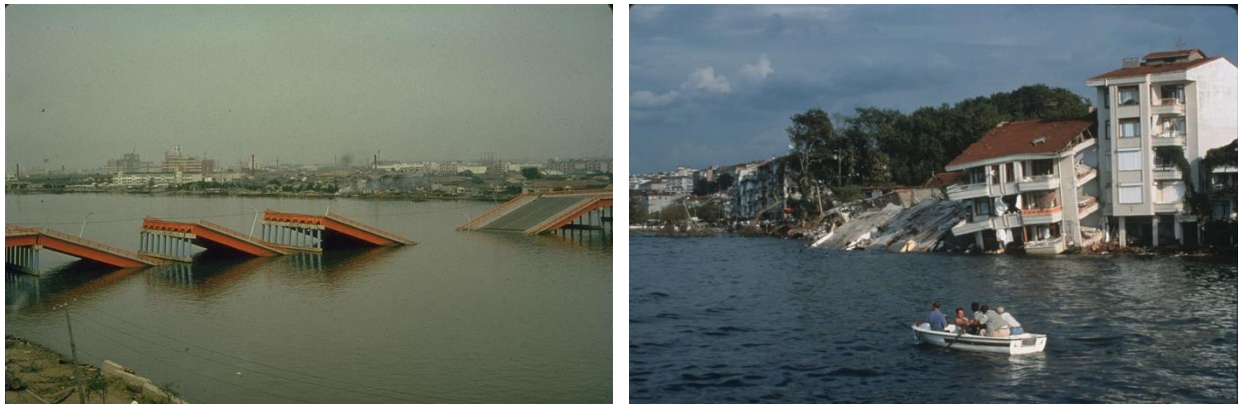
FIGURE 3. (left) Fallen bridge spans caused by lateral spreading during the 1964 Niigata earthquake. (right) Lateral spreading of waterfront properties during the 1999 Kocaeli earthquake.
