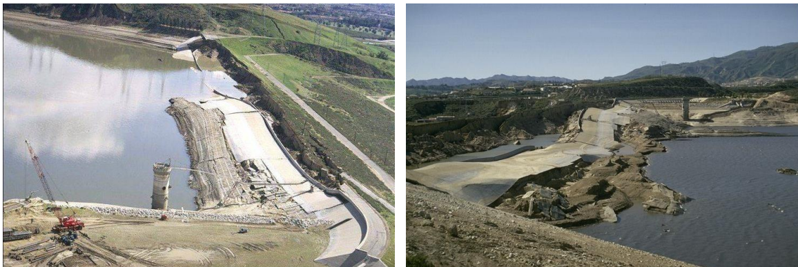
FIGURE 5. San Fernando Dam failure during 1971 San Fernando Earthquake.
