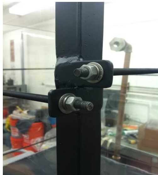
FIGURE 36. Close up of tie rod ends with bolting combination.
