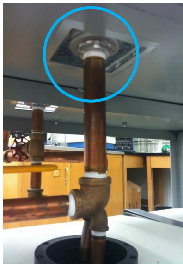
FIGURE 50. Inlet flow pipe connected to wall fitting.
